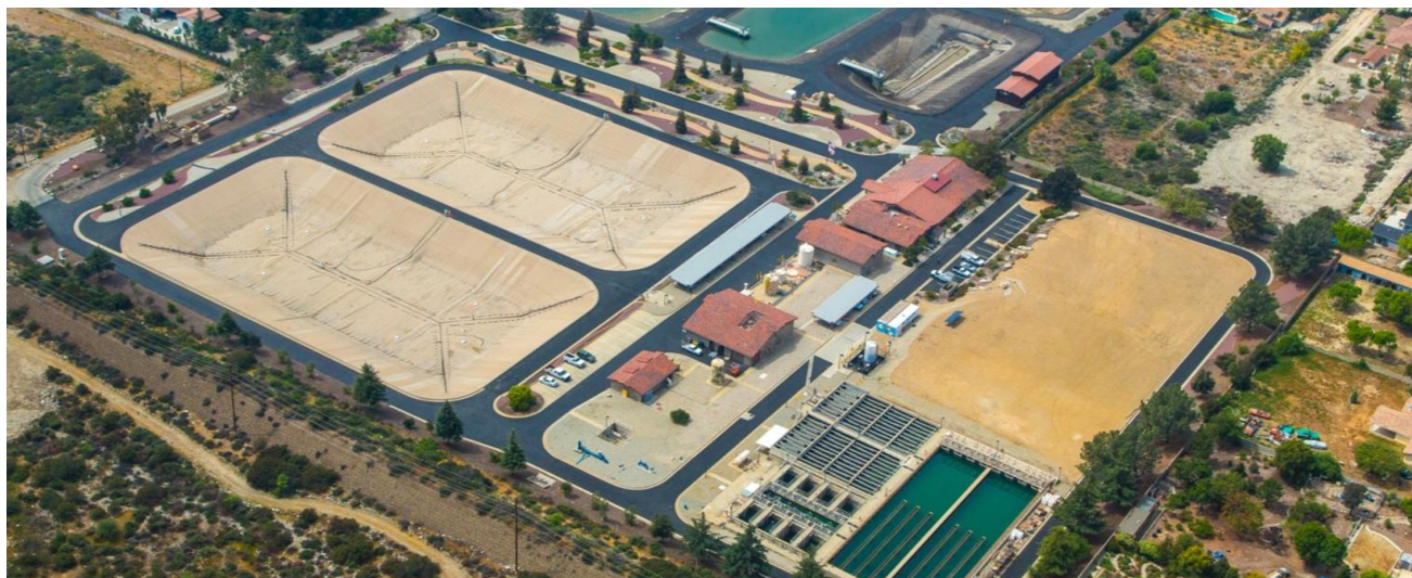
MIRAMAR TREATMENT PLANT
